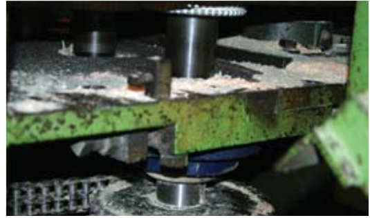
QM Bearings worked together with the mill to come up with a special secondary seal arrangement to keep the sawdust fines from contaminating the bearing, leading to increased bearing life.
